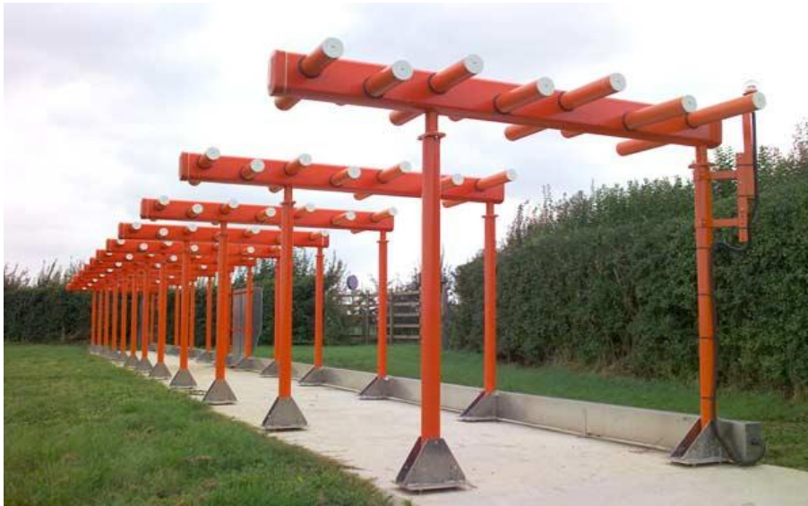
Localizer network using log periodic antennas
