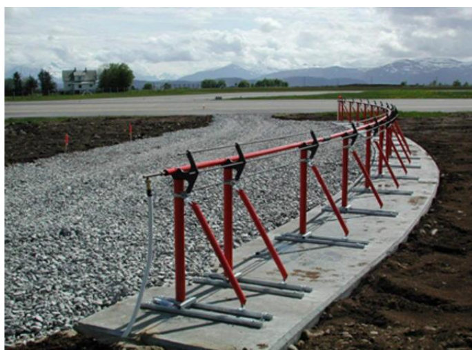
Close-up photo of the endfire system glide slope
